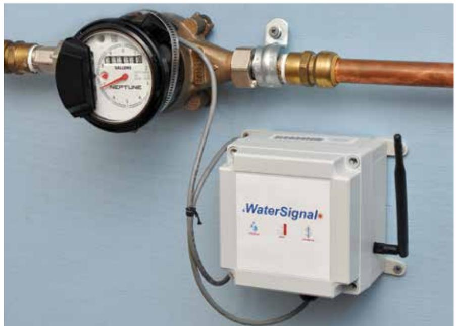
Wireless monitoring devices provide real-time water usage data, helping identify leaks quickly.
